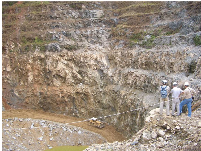
Figure 1 Refurbishment of open pit
