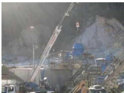
Figure 3 – Crusher being installed
