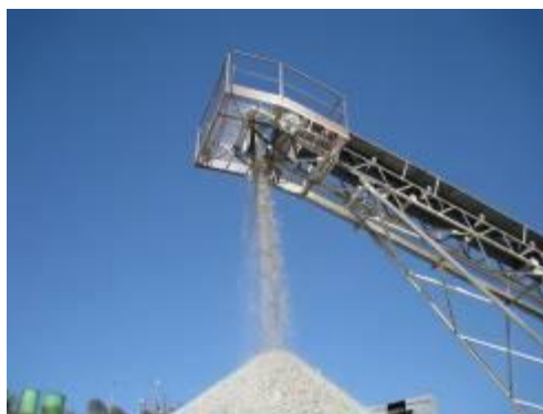
Figure 4 – Crusher fully commissioned
