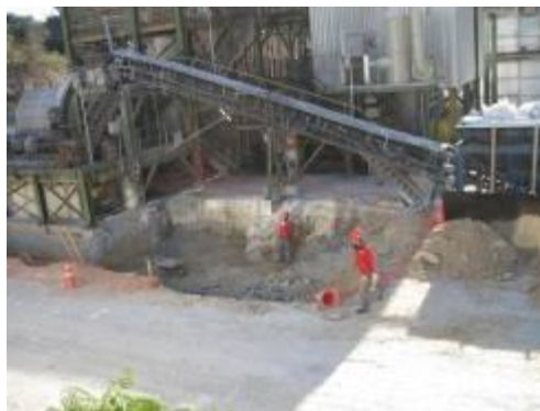
Figure 2 – Mill Foundations being put in place
