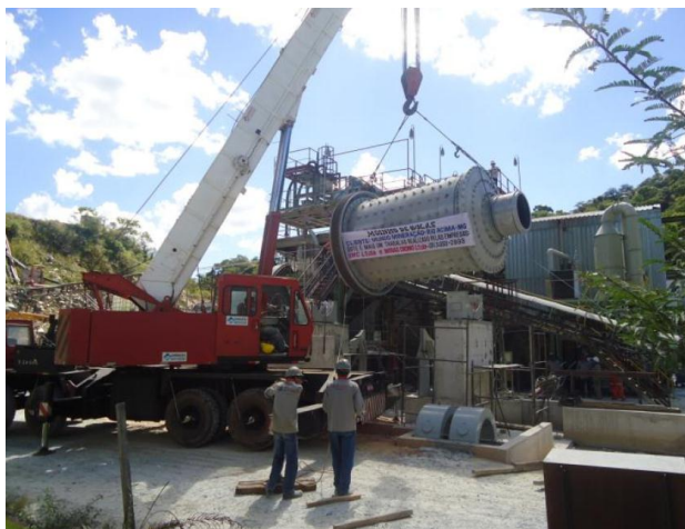
Installation of the new ball mill at Engenho
