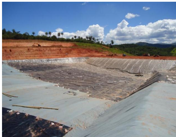
New Tailings dam with Stage 1 completed
